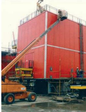
External Blast Wall Cladding
